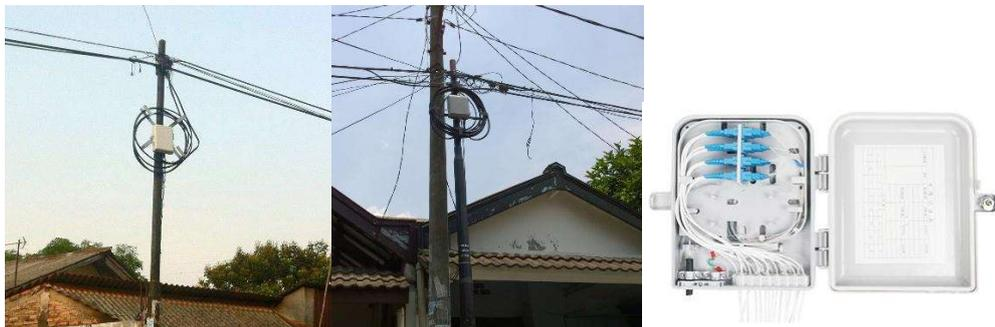
**Gambar 2. 10** ODP on the wall / pole dan ODP Pedestal
