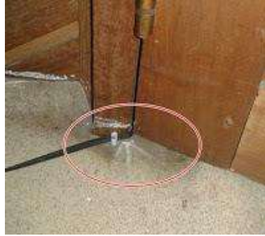
Gambar 2. 15 Kabel Fiber optic Tertimpa/tertindih Sumber : Data Penelitian (2021)
